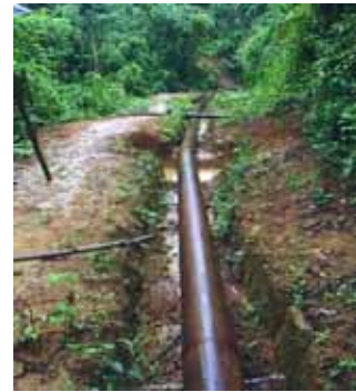
Laying of penstock
