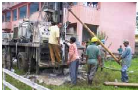
Drilling of tube well at The Govindajee Temple, Imphal.
