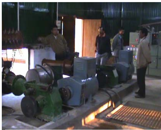
Trial run of Micro hydel being conducted
