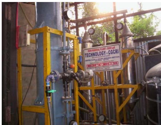
Machineries of iron removal plant installed
