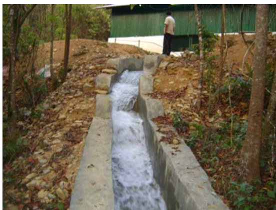
Flow of water in the tail race channel discharged by the turbine
