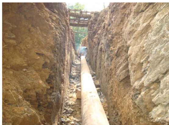
Penstock Pipes carrying water embedded inside the cross section of the rock cut to supply water to the turbine
