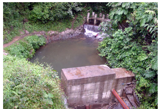
Fore bay tank and diversion weir
