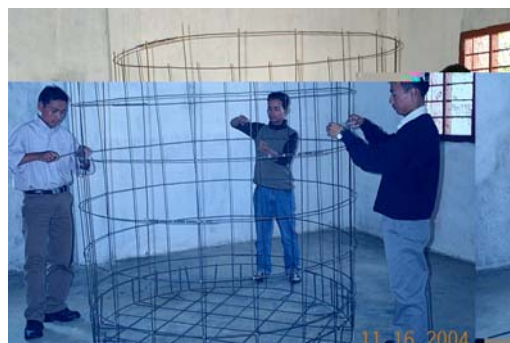
Fabrication of skeletal cage
