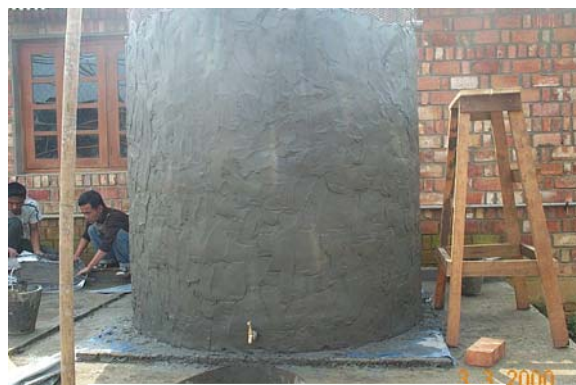
Plastering using cement mortar
